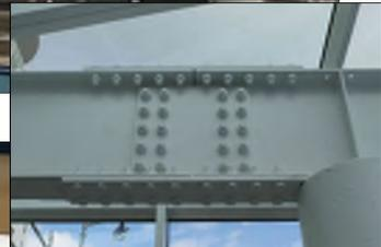
**New HSS Beam and a Typ. Splice to Connect New Structure to existing Steel Beams.**
