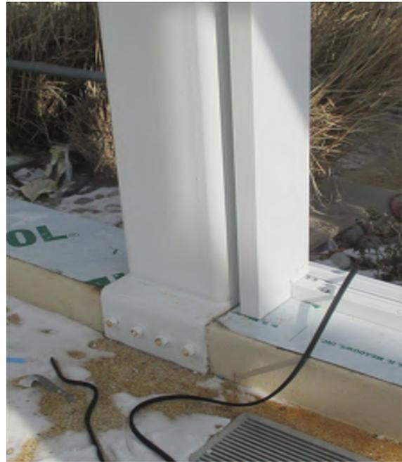
**Saddle Type Base Plate and Side by Side Double Moment Frames**
